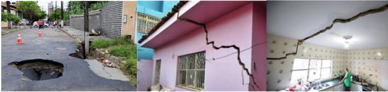
Figure 2, 3 and 4: Craters in the streets and cracks in buildings caused by earth moving. in the Pinheiro district. Source: Freitas (2019) [5].
