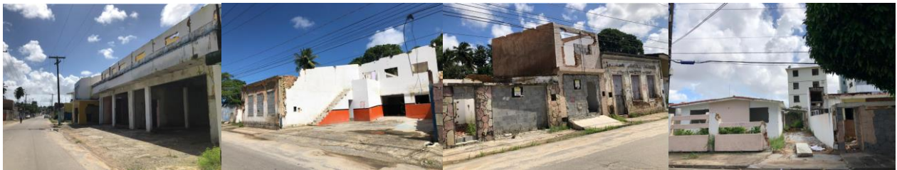
Figures 24, 25, 26 and 27: Empty and dilapidated buildings.
