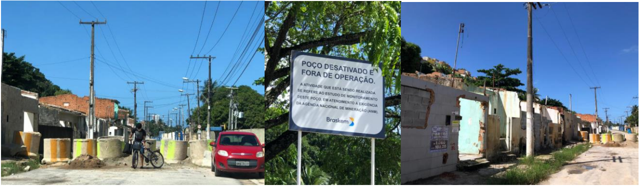
Figures 21, 22 and 23: Existing barrier in front of Braskem, there is no car passage.
