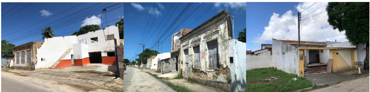
Figures 12, 13 and 14: Abandoned and dilapidated buildings in the affected neighbourhoods.
